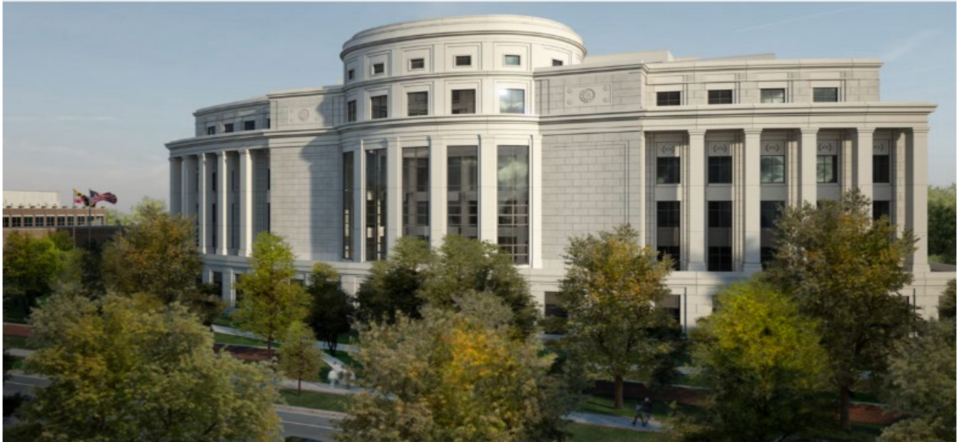
AERIAL VIEW FROM ROWE BLVD
