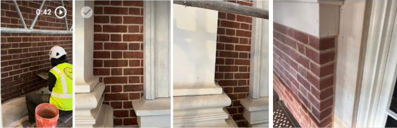
Pointing in process and restoration completed on various sections of wall
