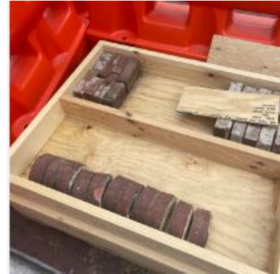
Retaining wall restoration has begun with selective deconstruction, salvage of materials for re-use and establishment of a temporary construction entrance
