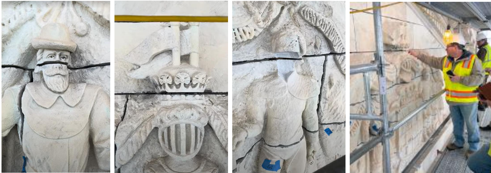
Fully prepped for restoration measures including stone dutchmen, crack grout injection, micro-pinning and pointing mortar
