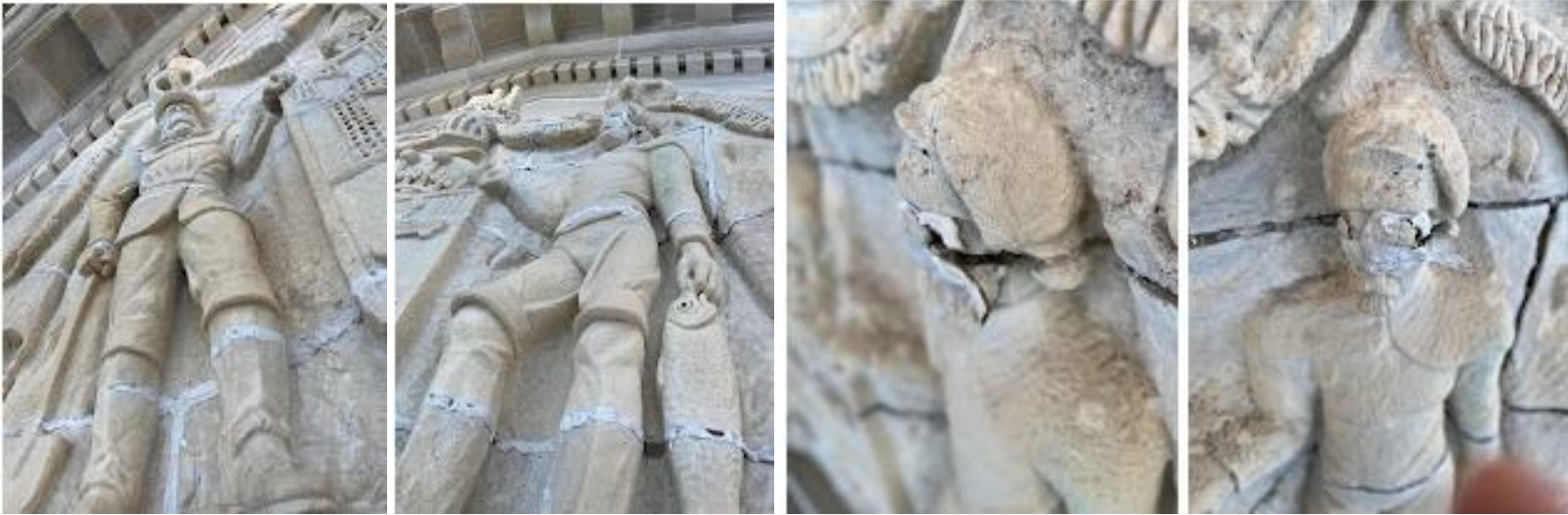
Existing condition of State Seal; deteriorated stone held together by failing (and inappropriate) caulk
