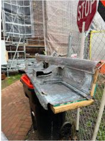
Cornice section w/ lead-based paint abated
