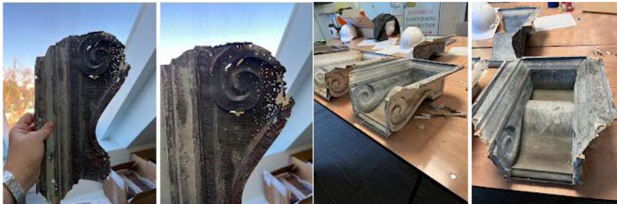
Metal cornice - condition of corbels
