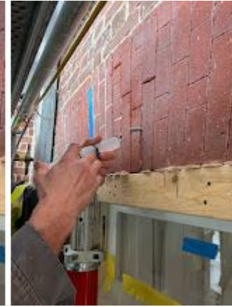
Micro-injection of lime-putty mortar using syringes
