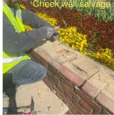
Retaining wall restoration has begun with selective deconstruction, salvage of materials for re-use and establishment of a temporary construction entrance
