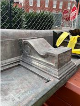
Cornice section w/ lead-based paint abated
