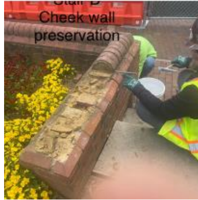
Retaining wall restoration has begun with selective deconstruction, salvage of materials for re-use and establishment of a temporary construction entrance
