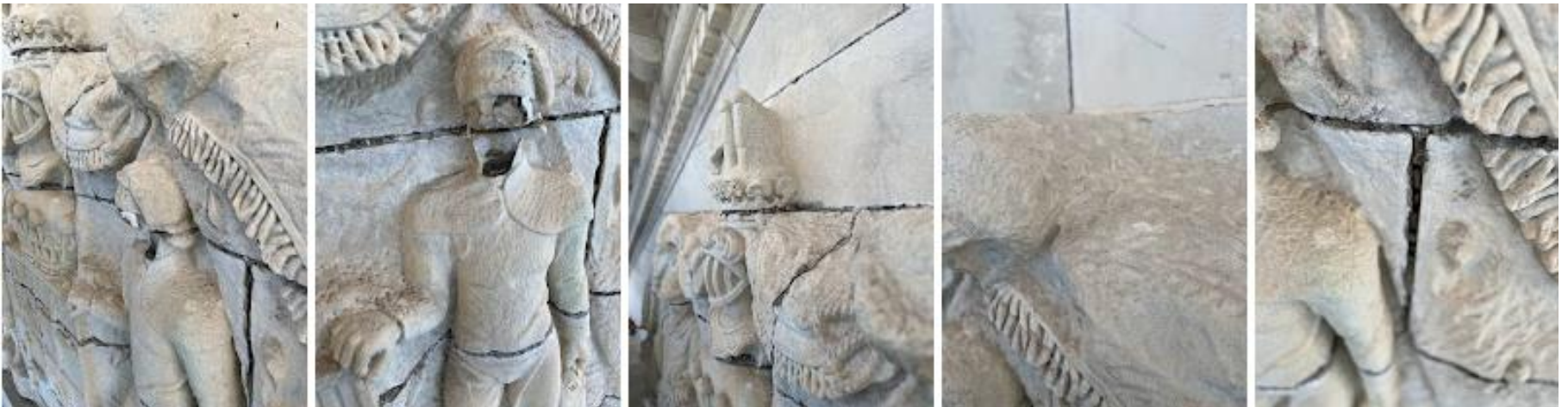
Inappropriate sealants and loose sections of stone removed; joints being prepped for removal of loose mortar
