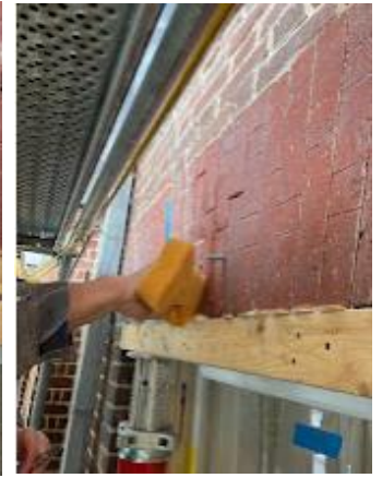
Micro-injection of lime-putty mortar using syringes
