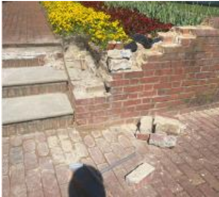
Retaining wall restoration has begun with selective deconstruction, salvage of materials for re-use and establishment of a temporary construction entrance
