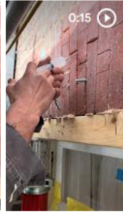
Micro-injection of lime-putty mortar using syringes
